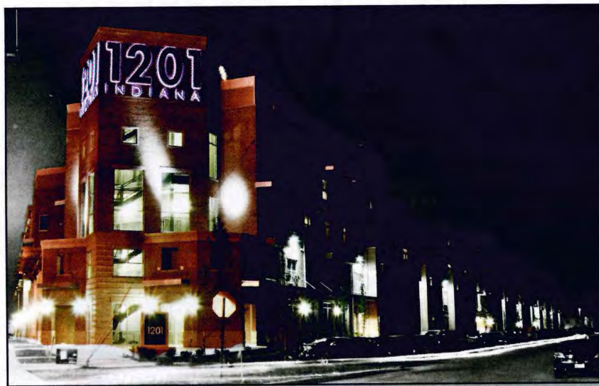
Harrison Street partnered with Trinitas Ventures to develop 1201 Indiana at Indiana University-Purdue University Indianapolis.
