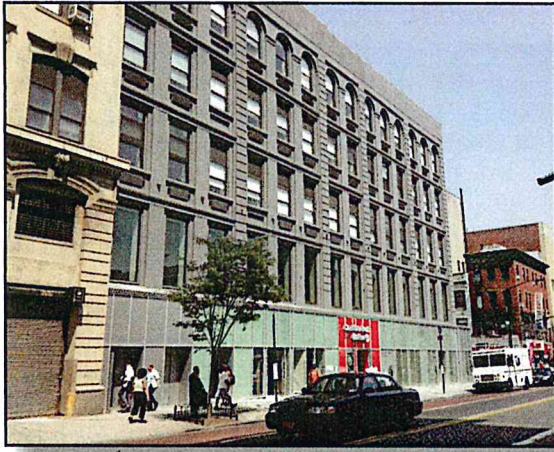
490 Fulton Street Serves Long Island University. It is a direct investment for Harrison Street.
